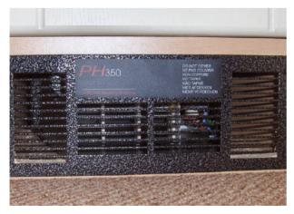
Where fitted, these are located within the plinths of wardrobes and kitchen base units. They are fan assisted electrically powered space heaters and are isolated by a fused spur or socket, and protected by an appropriately sized fuse. For safe operation please refer to the manufacturer's handbook provided with your holiday home or directly to the manufacturer's website. These
