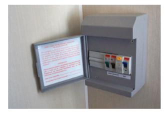
The consumer unit is usually installed in the main bedroom wardrobe. If the power fails check the RCD and breakers in the consumer unit. If they are not positioned as shown above in the photograph, then turn back on as shown above, i.e. with the switches located at the upper position. If the switch keeps tripping, contact your park or an approved electrician (NIC-EIC or similar).
